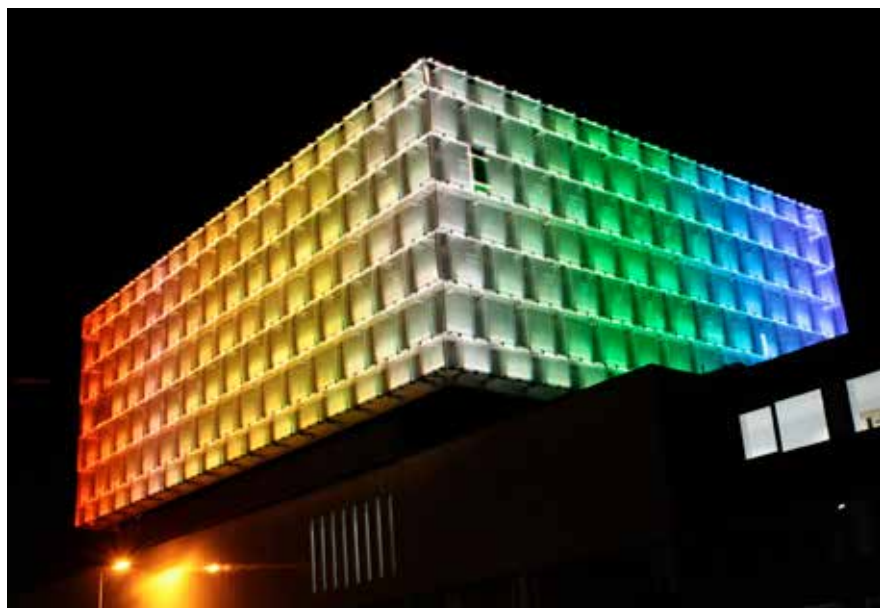
▲ University of Liverpool Faculty of Engineering building
