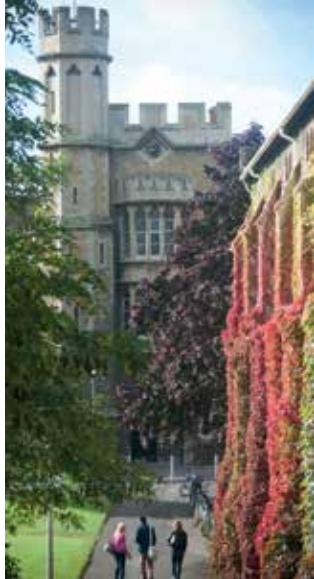
▼ Francis Close Hall campus
